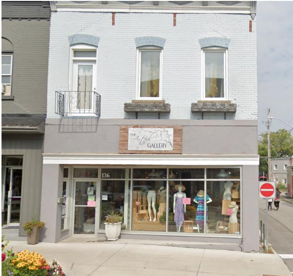
1. John Street North (Front Entrance)
