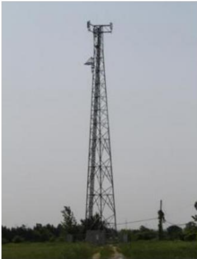
Figure 2- Example of Self Support Tower (Type S)
