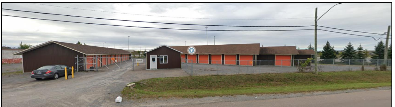
Figure 1 Streetview of 150 Staye Court Drive
