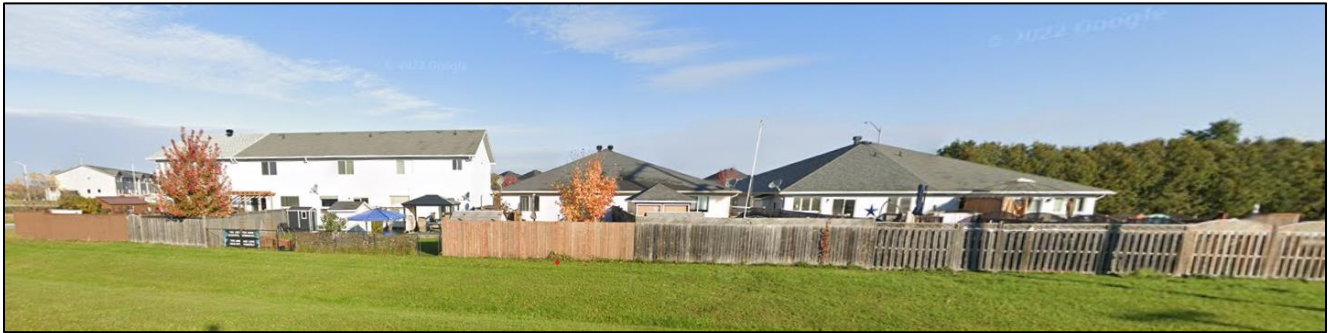
Figure 3 Rear yards of existing townhouses and semi-detached dwellings north of 150 Staye Court
