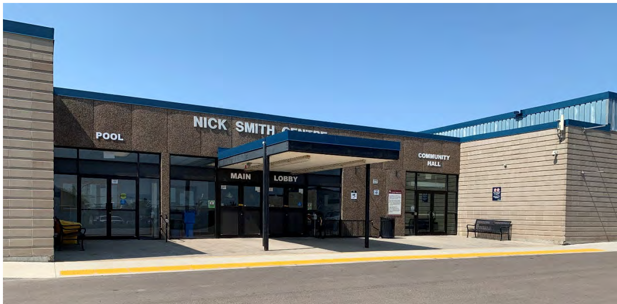
Figure 18 – Nick Smith Centre Entrance
