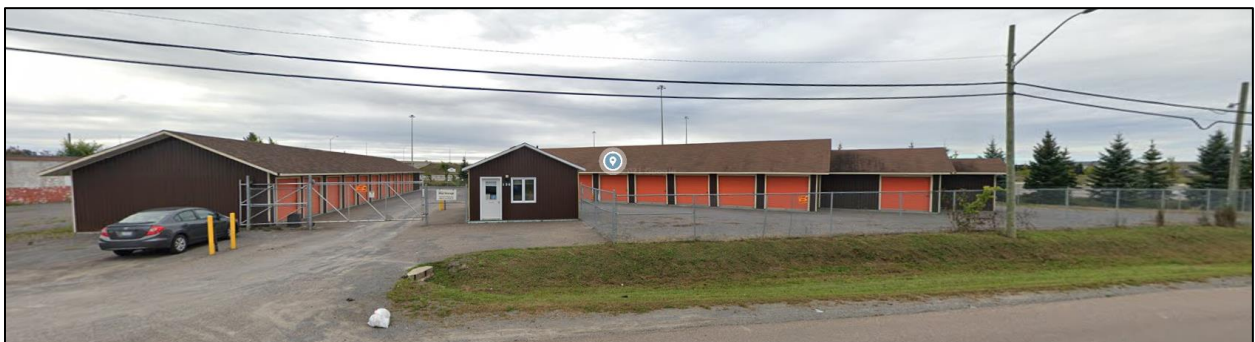
Figure 1 Streetview of 150 Staye Court Drive
