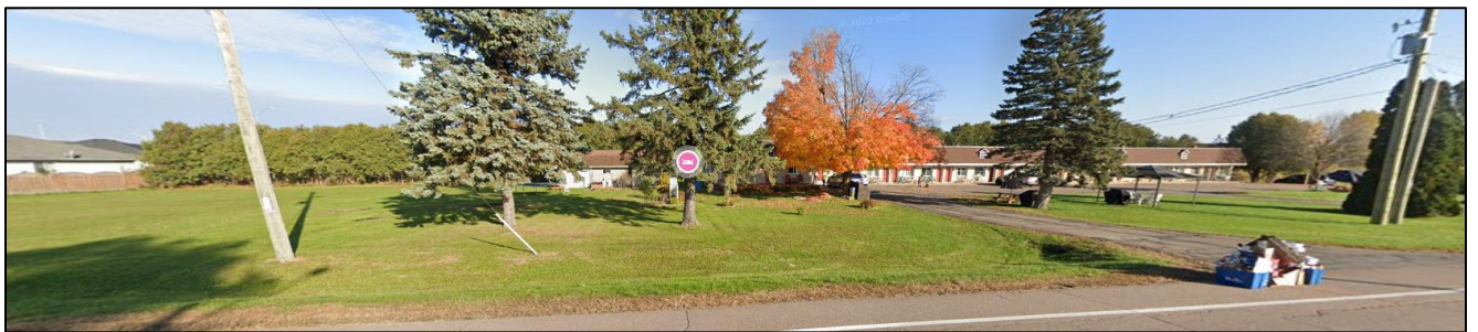
Figure 4 Streetview of the existing Country Squire Motel
