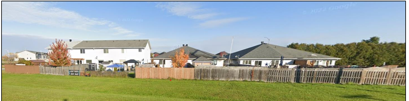
Figure 3 Rear yards of existing townhouses and semi-detached dwellings north of 150 Staye Court
