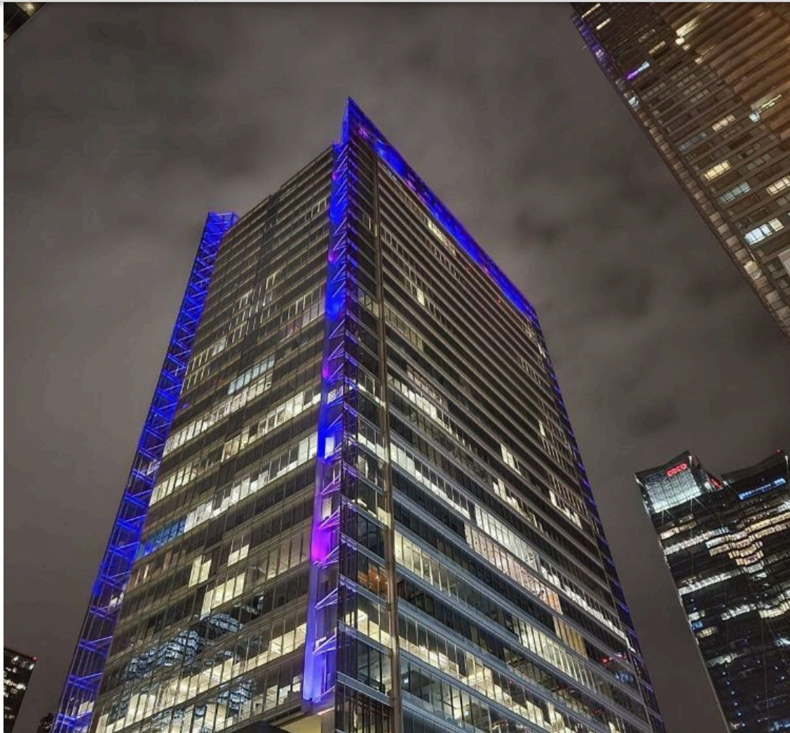
Telus Tower, 25 York Street, Toronto - photo provided by ODEN
