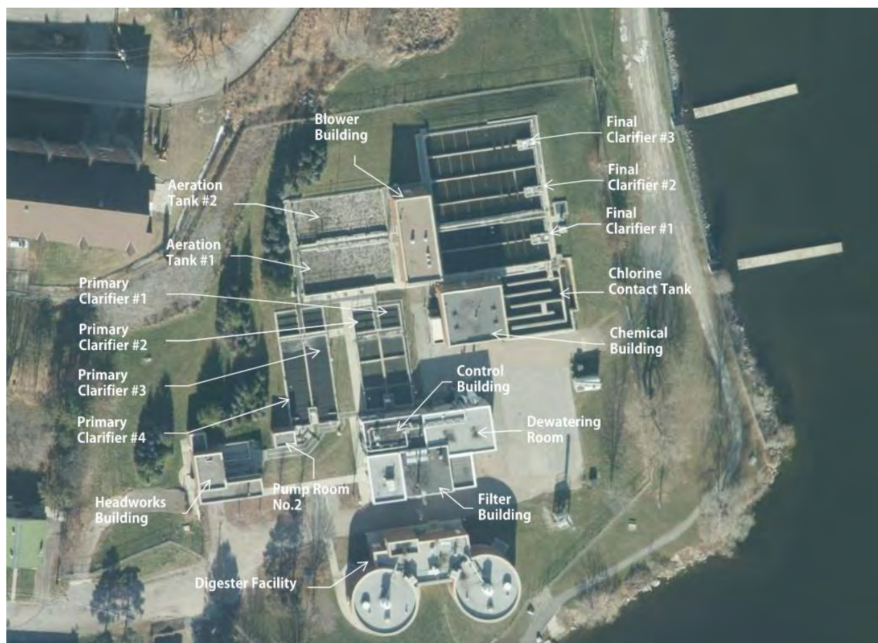
Figure 1: WPCC Aerial Photo
