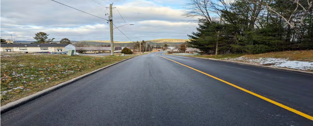
County Road 73 (Deep River Road), Town of Deep River
