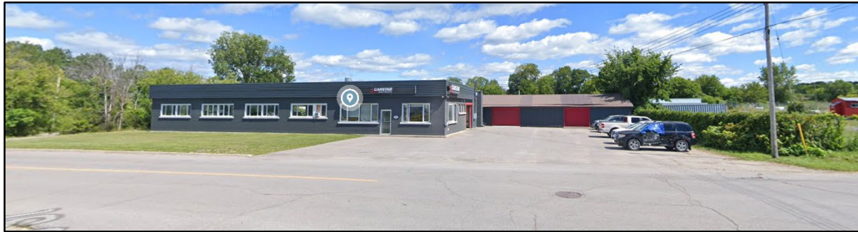
Figure 3 Streetview of 100 McNab Street
