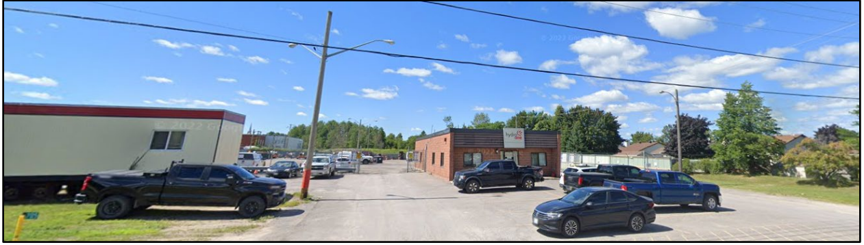
Figure 5 Streetview of 205 McNab Street
