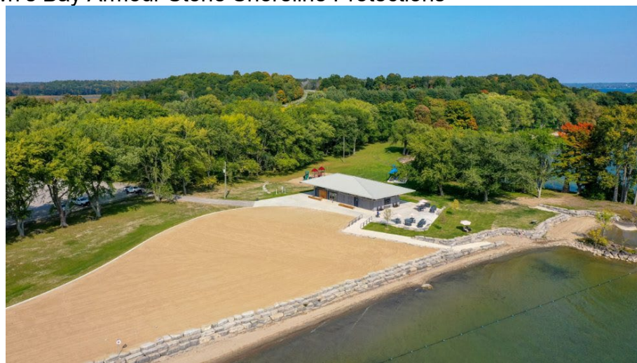
Figure 6: Brown's Bay Armour Stone Shoreline Protections
